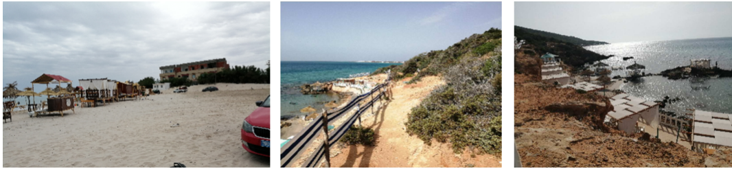
Figure 53: Installation of straw huts along the coastal fringe of Sidi Ali el Mekki.
