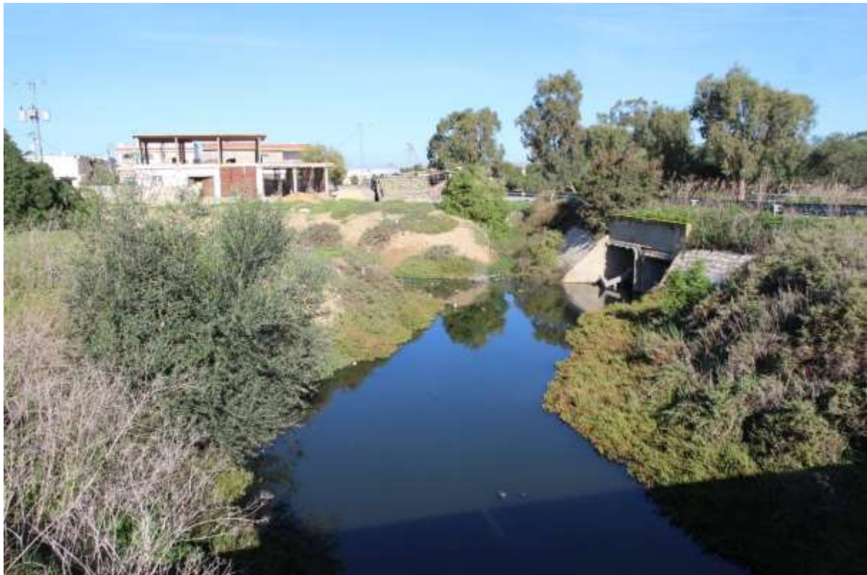
Figure 8 Saline canal confluence south of Aousja. Photo: © R. Lansdown
