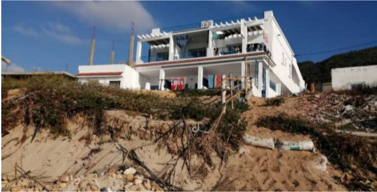
Figure 12 Building construction on the base of the hill, along the coastal fringe. Photo: © R. Lansdown
