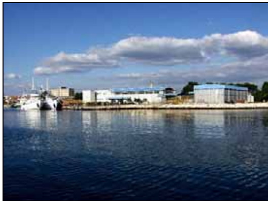
Marituna's processing plant and storage facilities
