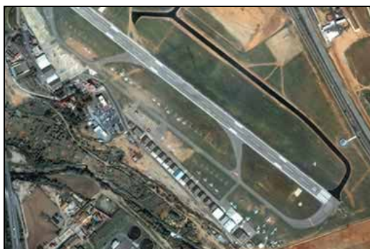
Sabadell airport, Spain.
