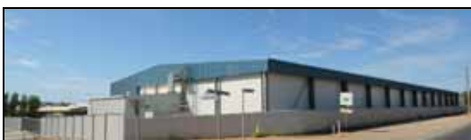
Outside freezers at Windsor Avenue, Port Lincoln
