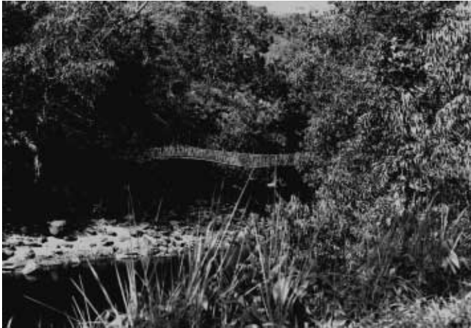
Figure 1.7 A few such hanging rattan bridges are still in use
