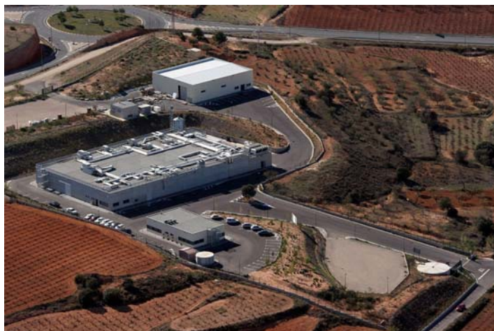
Mediterranean fruit fly mass-rearing facility, Caudete de las Fuentes, Valencia (Spain), with a production capacity of 500 million sterile males per week.
