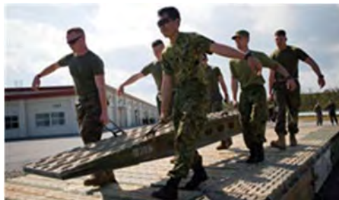
Assembly of a Medium Girder Bridge (MGB)
