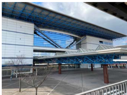
Main hall entrance
