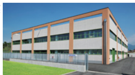
Mesdan-Lab new plant
