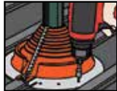
5. Fasten Retrofit to roof
