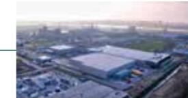
Accoya® Arnhem Plant 50% capacity increase completed in year
