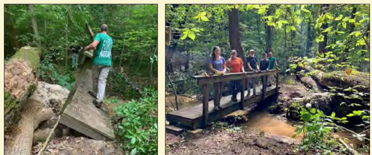
On the bridge l to r: CCC Intern Nicole Stevens, Former CCC Intern Rachel Delbow, Volunteers Jeff Buyer, Paul Blayney, and Kevin Donahue. Kevin is on the bridge in the before photo.
