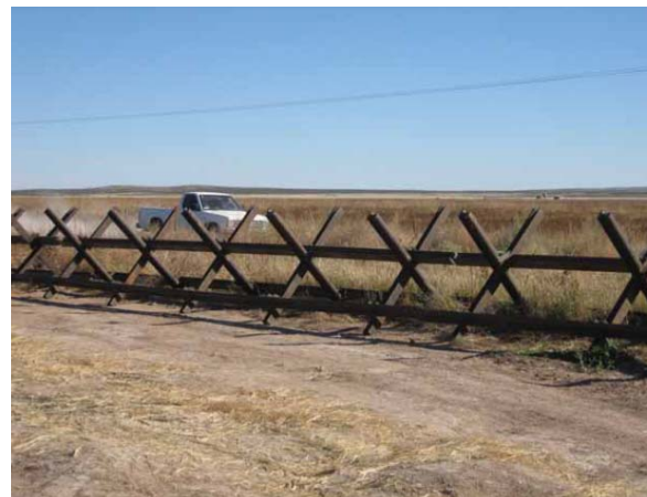
Photograph 2-2. Vehicle Fence (Normandy-style).
