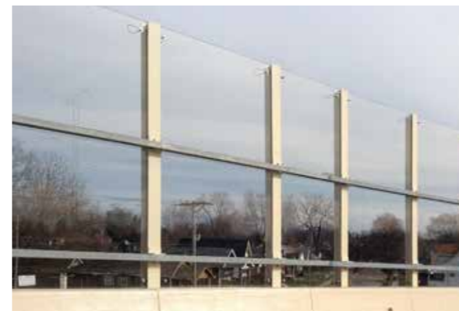
ACRYLITE® Soundstop GS CC TL4 System at Exit 19 on I-475 in Toledo, OH
