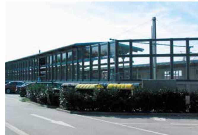
Noise barrier, Railway station Baden Baden PLEXIGLAS® Soundstop GS CC R. Kohlhauer GmbH
