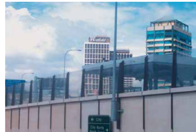
Noise barrier, Eastern Distributor, Sydney PLEXIGLAS® Soundstop XT and GS CC Leighton Constructions
