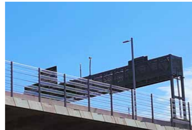
Wind screen, Mersey bridge, Liverpool PLEXIGLAS® Soundstop GS Liverpool
