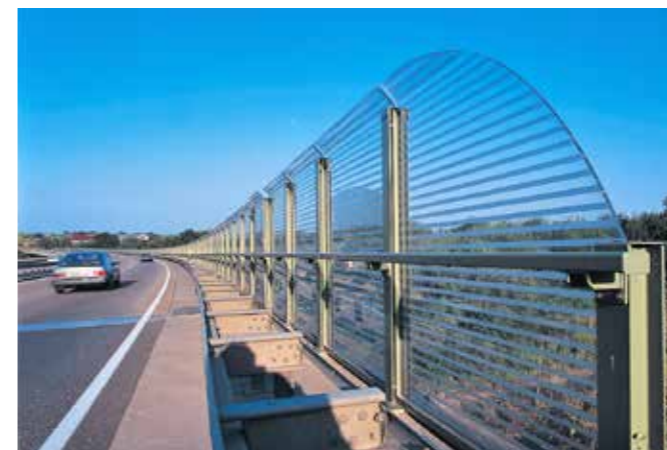
Noise barrier, Eltville PLEXIGLAS® Soundstop XT
