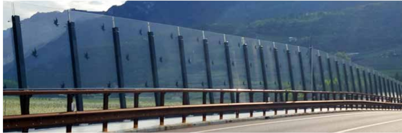
Noise barrier, Highway Trento Sud Flyover PLEXIGLAS® Soundstop GS CC 20 mm, Clear Trento Sud Flyover
