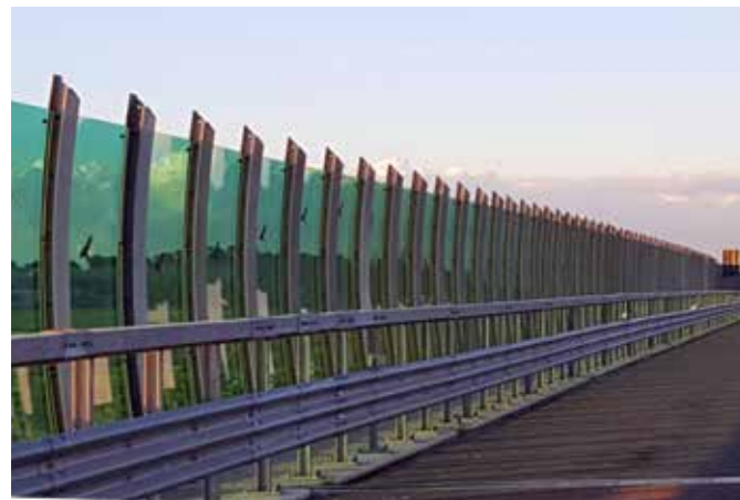
Noise barrier, Highway Valdastico Sud PLEXIGLAS® Soundstop XT 20 mm, Spring Green Valdastico
