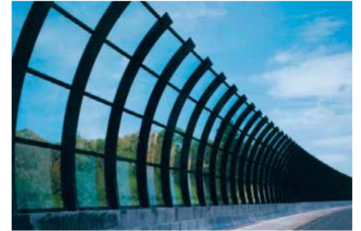
Noise barrier, M5, Melbourne PLEXIGLAS® Soundstop John Holland
