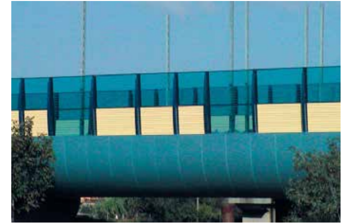
Noise barrier, high-speed section Rom-Neapel PLEXIGLAS® Soundstop XT Saico Spa, Arezzo
