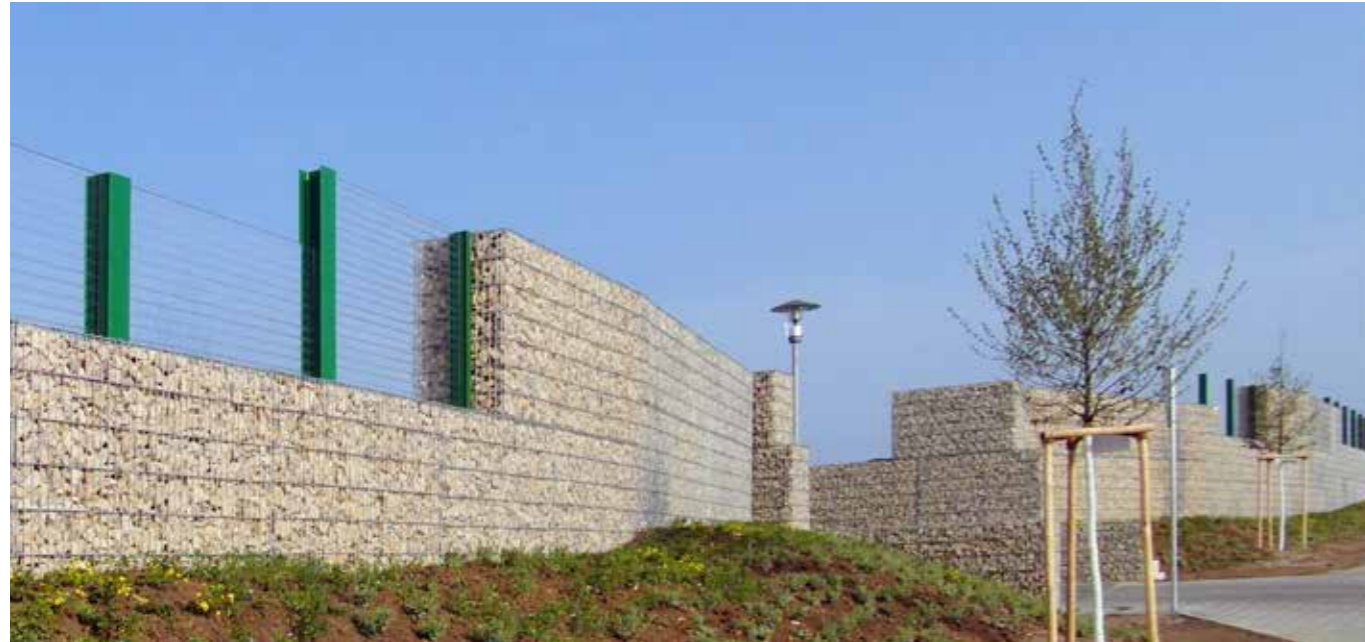
Noise barrier, Pollenfeld PLEXIGLAS® Soundstop XT BirdGuard, 20 mm
