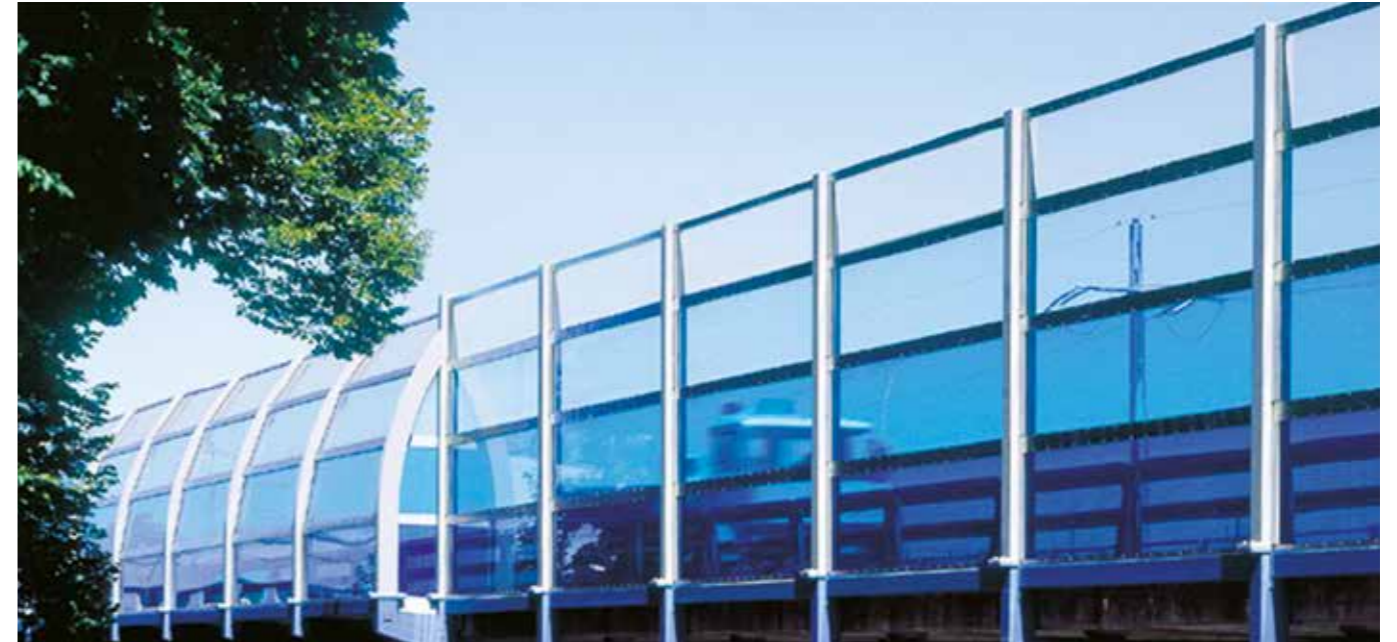
Noise barrier, Highway N1, Morges West, Kanton Waadt PLEXIGLAS® Soundstop GS Usine des Jurats S.A.
