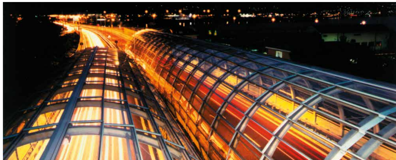
Tunnel entrance, Monte Barro, Lecco PLEXIGLAS® Soundstop XT Tubosider ITALIANA S.p.A.
