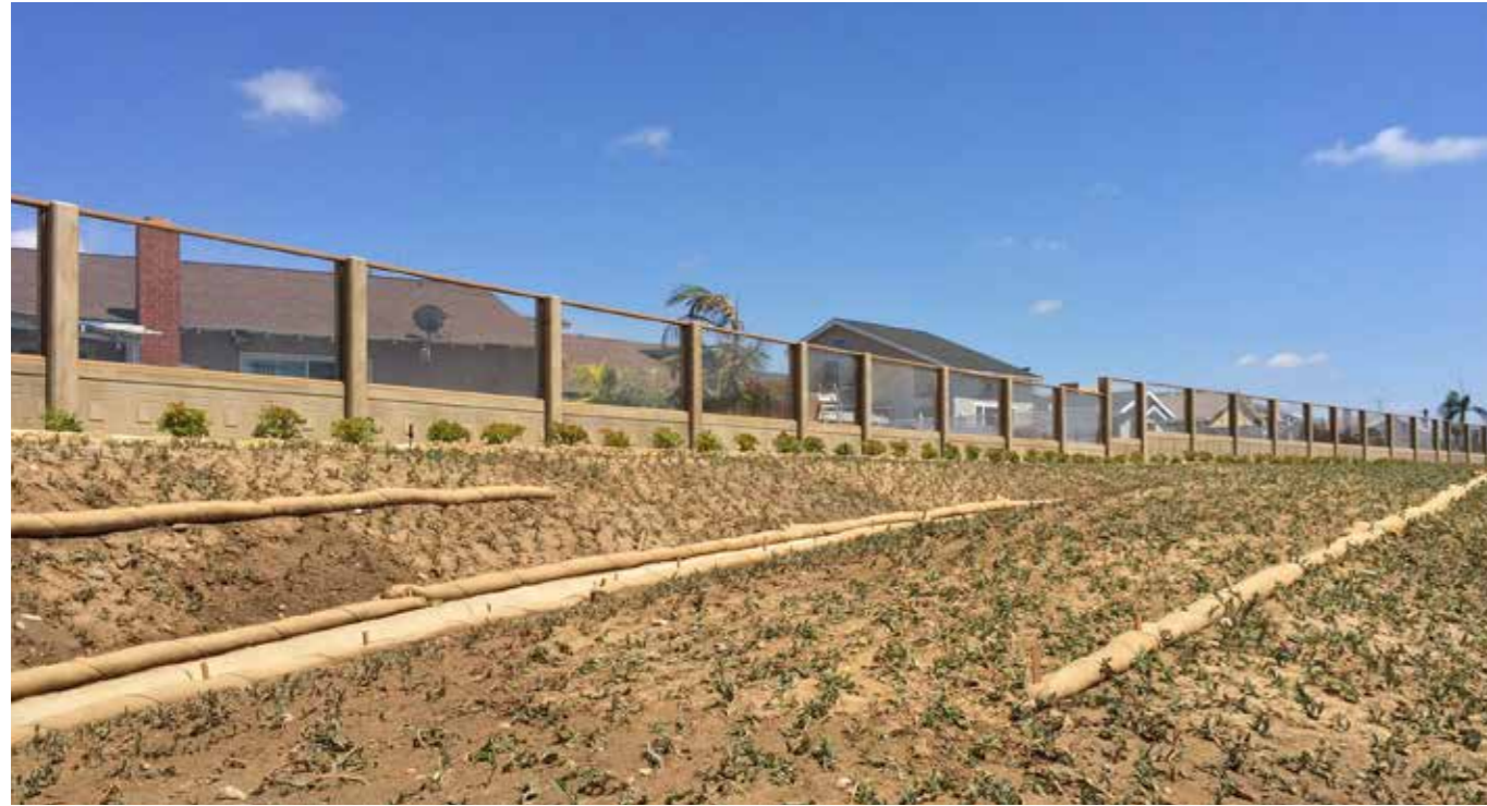
ACRYLITE® Soundstop Ready Fit System with anodized bronze framing near Telegraph Canyon Road off the I-805 Freeway in Chula Vista, CA
