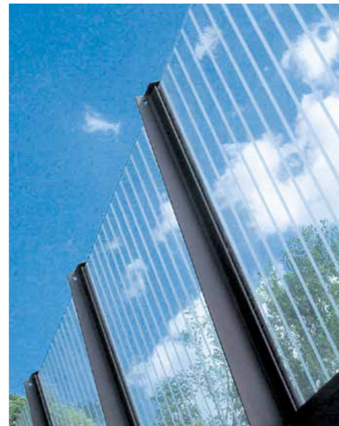
Noise barrier, Highway N1, Morges West, Kanton Waadt PLEXIGLAS® Soundstop GS Usine des Jurats S.A.
