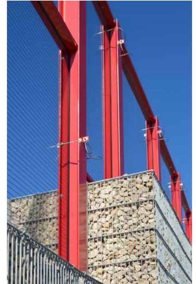
Noise barrier, Pirmasens PLEXIGLAS® Soundstop GS CC, 15 mm
