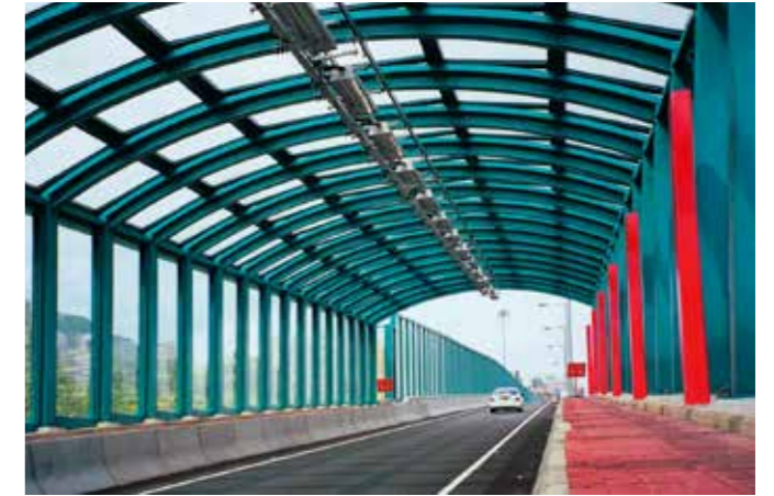
Inside view of noise control tunnel Eastern Corridor PLEXIGLAS® Soundstop GS CC and GS Active Way Ltd.
