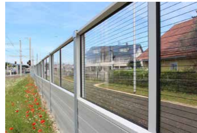
Noise barrier, regional tram Traun test track PLEXIGLAS® Soundstop GS CC Forster Metallbau Gesellschaft m.b.H. Traun
