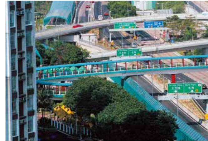
Noise barriers, noise control tunnel Eastern Corridor PLEXIGLAS® Soundstop GS CC and GS Active Way Ltd.
