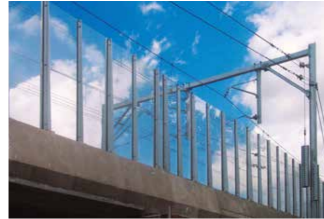
Noise barrier, Parramatta Rail Link, Sydney PLEXIGLAS® Soundstop GS CC Ingal Civil Products
