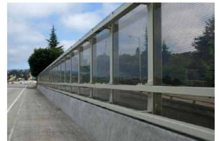
ACRYLITE® Soundstop GS CC TL4 System on I-580 just before Foothill Blvd. in San Leandro, CA
