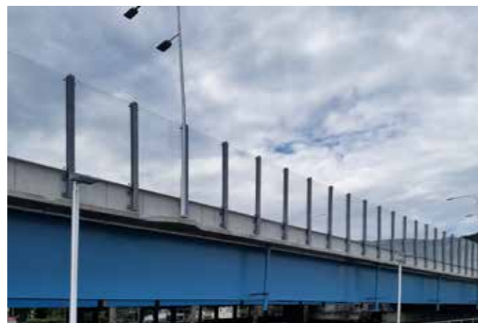
ACRYLITE® Soundstop GS CC Structure Mounted System on the Governor Mario M. Cuomo Bridge, Tarrytown, NY
