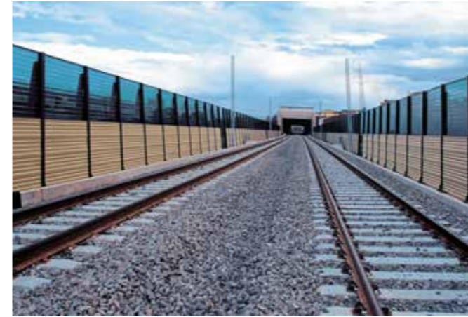
Noise barrier, high-speed section Rom-Neapel PLEXIGLAS® Soundstop XT Saico Spa, Arezzo
