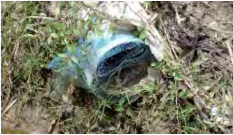
Photo G. Example of inefficient screen at the inlet of a pond (Liberia) [© Y. Fermon].
