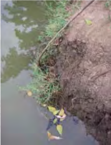
Photo F. Dikes. On left: Slope badly constructed, destroyed by erosion (DRC)[© Y. Fermon]; On right: Construction (Ivory Coast) [© APDRA-F](CIRAD).
