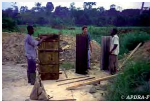
Photo I. Mold and monks (Guinea). On left: The first floor and the mold; On right: Setting up the second floor [© APDRA-F] (CIRAD).
