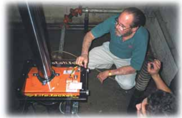
LifeJacket installs above the cylinder head. It is shown above with arms open in the "operate" position
