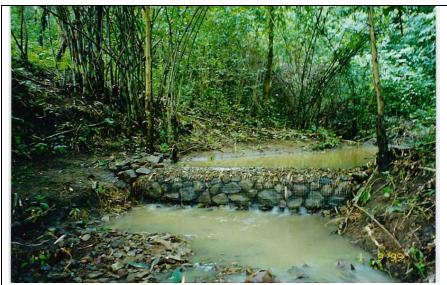
Figure 19: Example of a rehabilitated weir.
