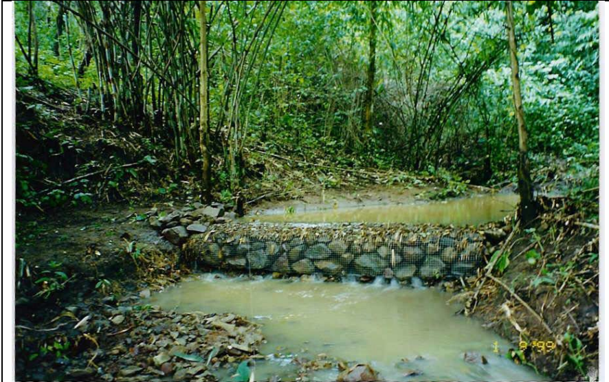
Figure 19: Example of a rehabilitated weir.
