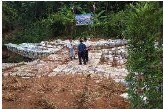
Living Check Dam construction
