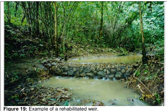
Figure 19: Example of a rehabilitated weir.
