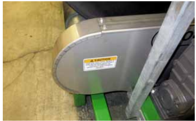
Cover Installed (Typical)
