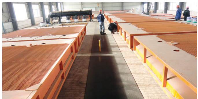
Ring furnace construction at our Yangquan (China) site.
