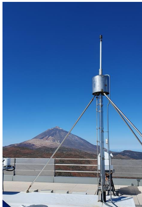
Figure 5.1. Sample inlet for reactive gas measurements located on top of the Izaña Observatory technical tower in front of the Teide volcano.
