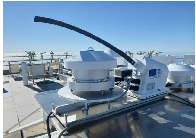
Figure 10.4. The EKO RSB spectroradiometer installed at IZO.
