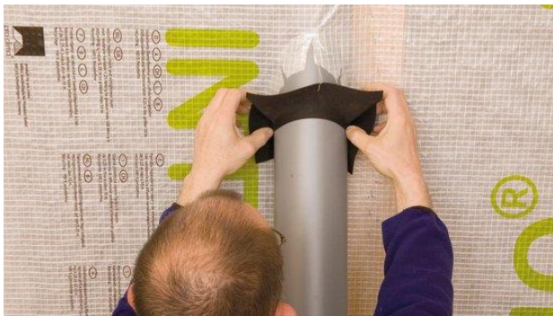
1. Pull the grommet over the pipe and align it
