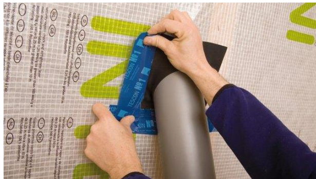
2. Stick the grommet and rub it firmly in place
