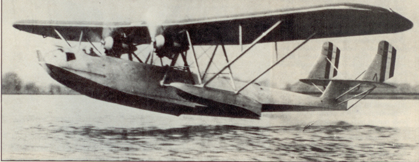
The Consolidated XPY-1 Admiral was the Navy prototype of the civil Commodore airliner. Although designated a patrolplane, it could carry bombs and torpedoes. Built in 1928, it had a gross weight of 13,500 pounds, a top speed of 120 mph and open cockpits for the pilot and bombardier.
