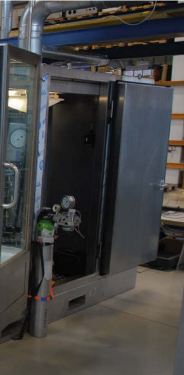
ABOVE: A test stand under construction
