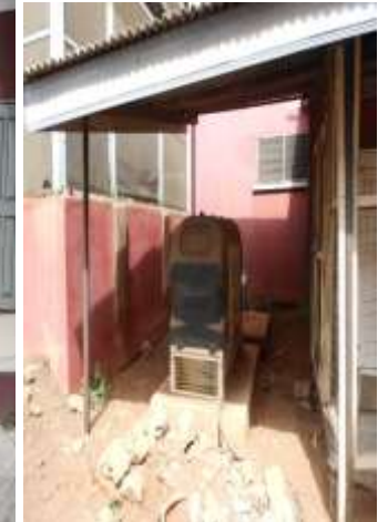
Relocation Generator Set 2
