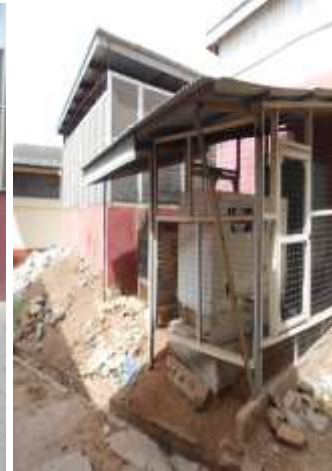
Relocation Generator Set 1
