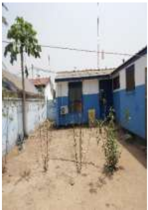
Back Section of Building
