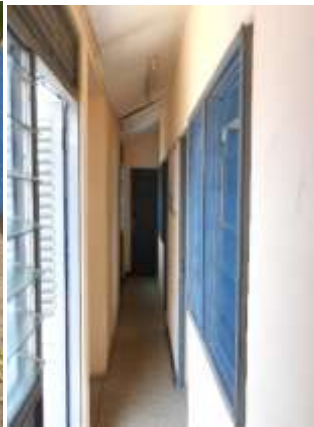
Interior Corridor Features
