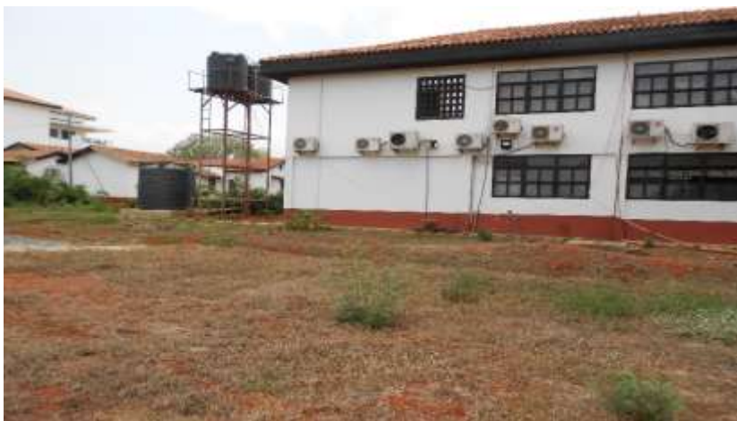
Back of the Existing Biotechnology Centre Building
