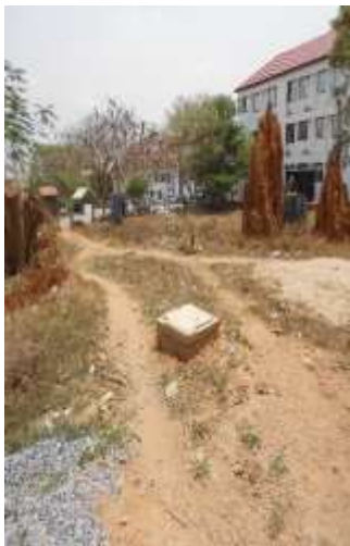
Sewage Line Chamber Presence
