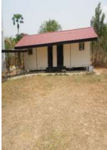
Relocation of Metal Container
