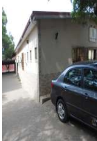
Partial Demolition (Animal Hse Bldg)
