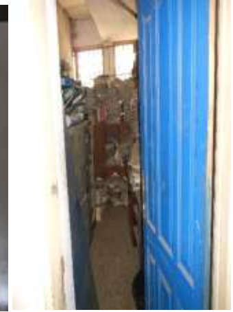
Old Storage Room
