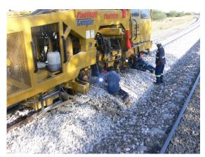
Photo 7.8.1 - Broken rail between Erundu and
