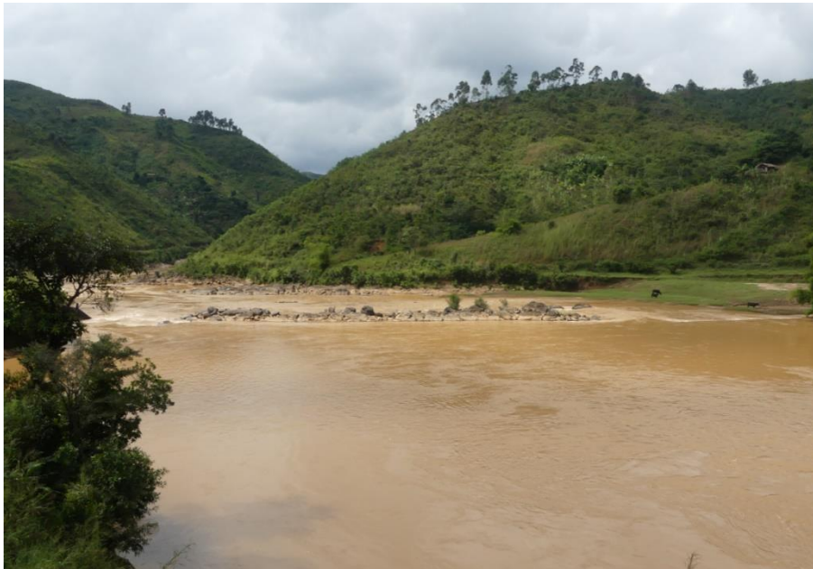
Figure 72 – Calm Diversion Bays Interspersed with Natural Sills Downstream from the Plant
