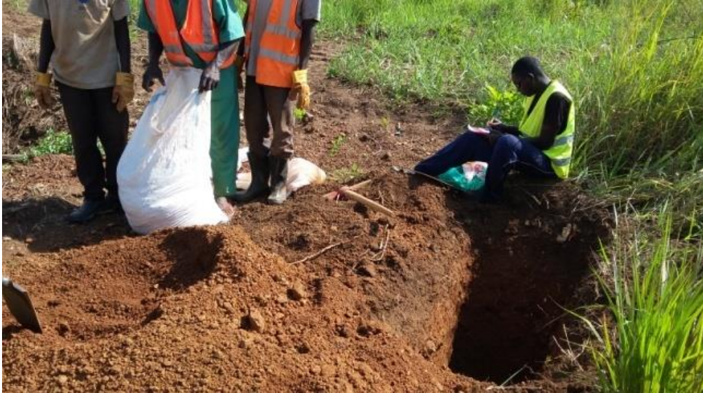
Plate 7: Borrow Area Test Pit Investigation and Sampling in the project area
