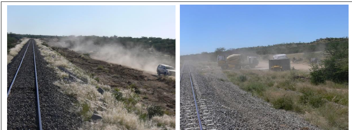
Photos 5.2.1-1 & 5.2.1-2 – Dust from maintenance vehicles operating within the servitude
