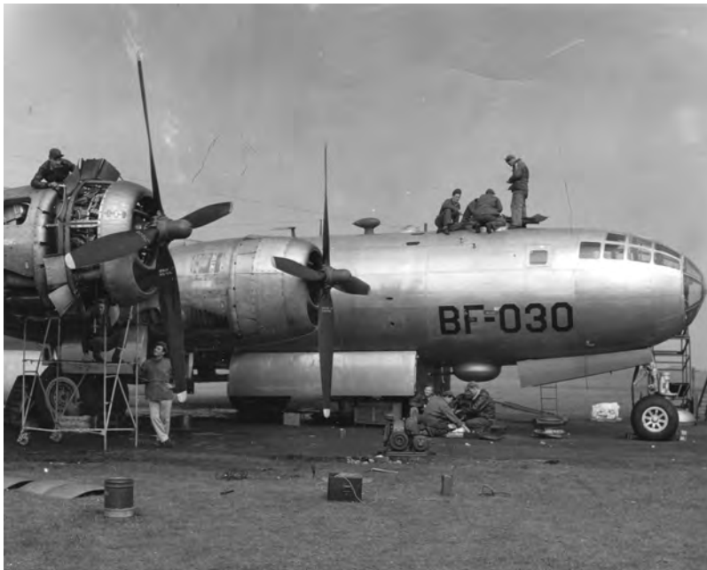
USAF B-29 ground crew personnel performing 100-hour inspection at RAF Scampton, 1948.
