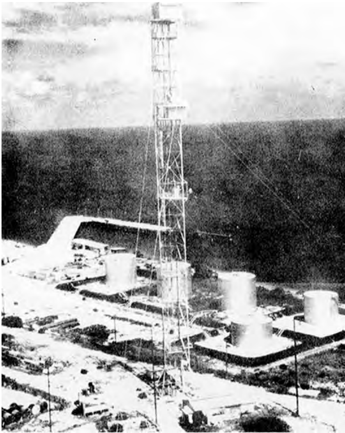
Figure 21. 300-foot instrumentation tower, Parry Island (Site Elmer) 1961. (USAF)
