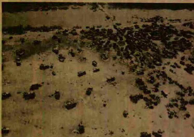
Air Photo Showing Result of Destruction of a Bridge During Encirclement Battle of Smolensk (1941)
