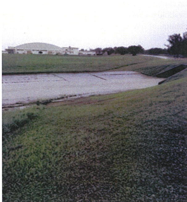
Figure 15: Photograph taken during stormwater outfall monitoring on 22 June 2020. (Tab W-20)
