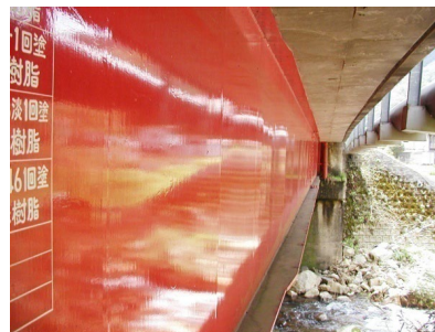
Bridge pier with Lumiflon coating (21 years-old)
