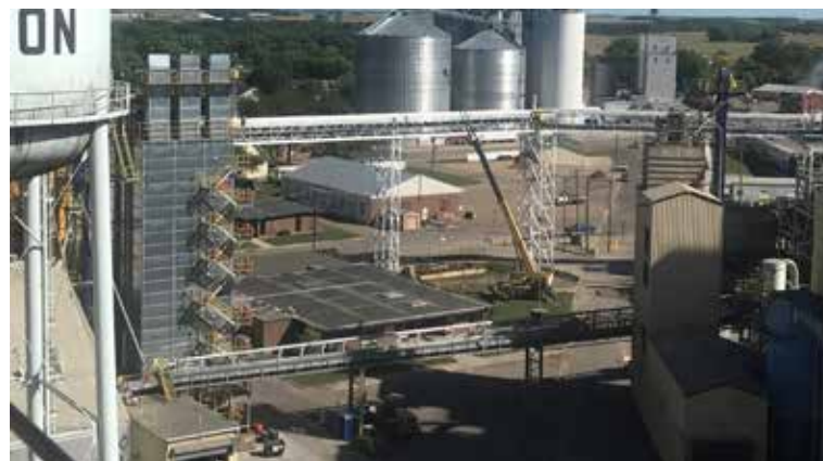
New conveyor bridges have been installed as part of an upgrade at the AGP soybean processing facility in Dawson, Minnesota.
