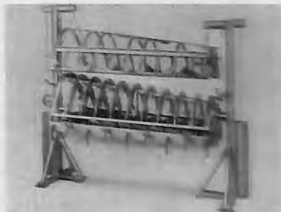
TWIX made tool for Routing, Drilling and Assembly of a Turtle Deck. (6' long, 4' high, 8" wide)
