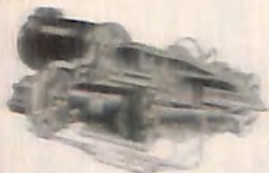
40 HP turbine driven unit, supplying electricity and hydraulic power.
