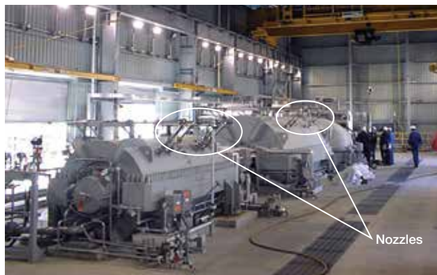
▲ Figure 5. Centrifugal compressors in ethylene plants come in varying configurations and can handle large volumes. Photo courtesy of Elliot Group.
