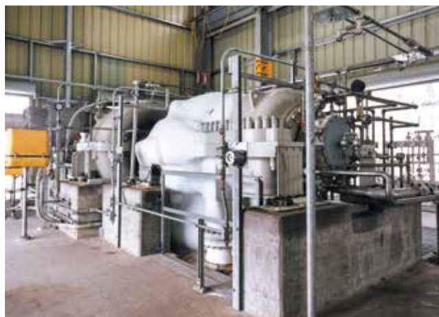
▲ Figure 11. In existing plants, refrigeration compressors are easy to find because they are covered in frost. Photo courtesy of Elliot Group.
