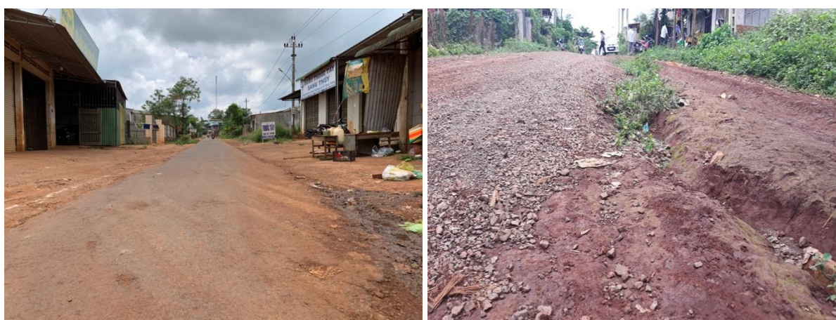
A concreted inter-village road in Cu Hriet village, Cu Pong commune
