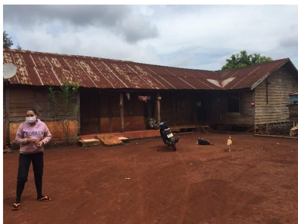
Semi-permanent, dirt floor, wood walls and roof
