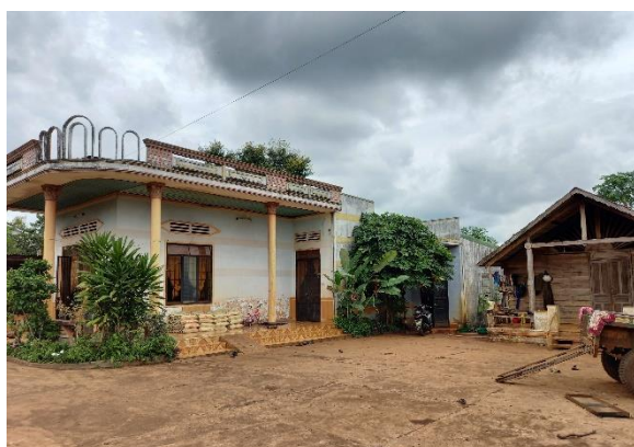
Permanent house in good conditions built next to a stilt house
