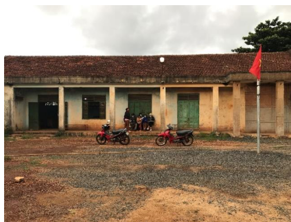
Cultural house in Ea Kung village
