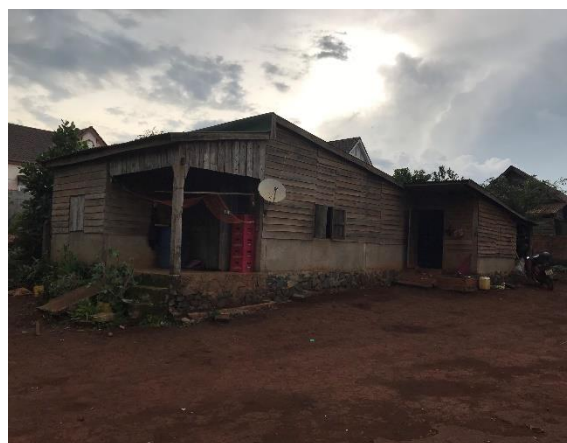
Semi-permanent house with cement floor, wood walls, and wood or tin roof
