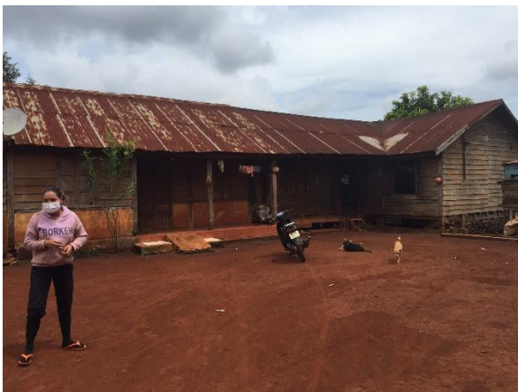
Semi-permanent, dirt floor, wood walls and roof
