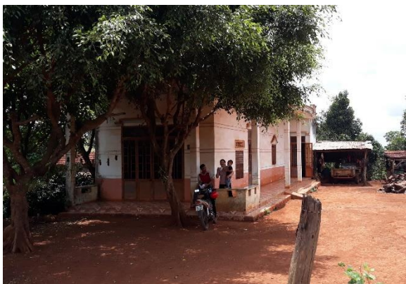
Permanent house with cement floor, tin or tile roof
