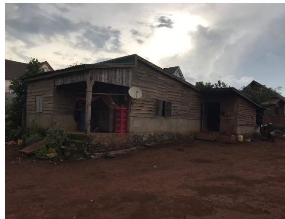
Semi-permanent house with cement floor, wood walls, and wood or tin roof
