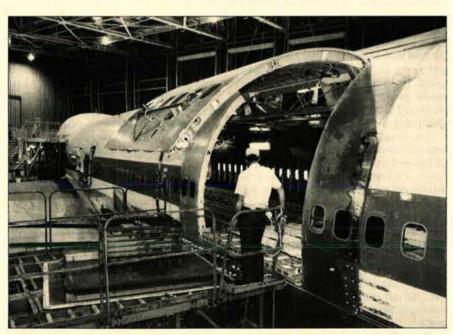
The first Boeing 747 to be converted to Civil Reserve Air Fleet (CRAF) configuration, shown here during conversion at the Boeing Military Airplane Co. plant, has been delivered to Pan American World Airways.
