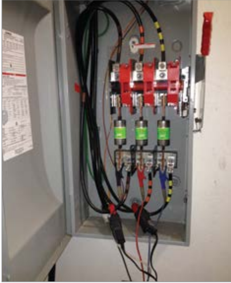
Figure 1: Using CTs is an effective method for recording kW.
