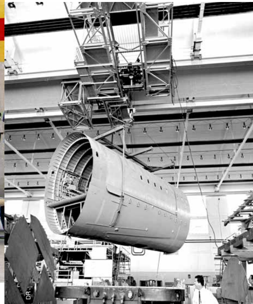
Shaft section 12 weighed 2.5 tonnes once equipped.
