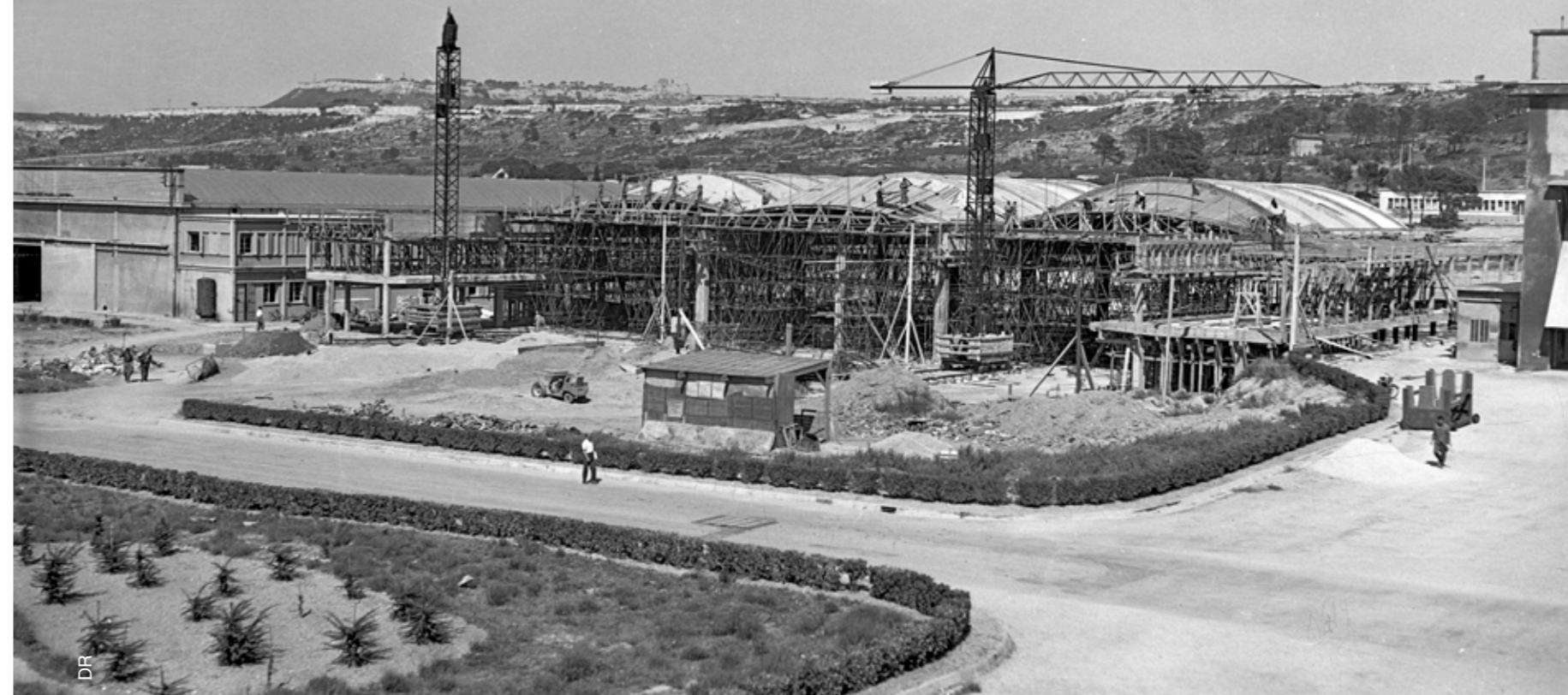
Construction of building L (upper factory) in September 1957.
