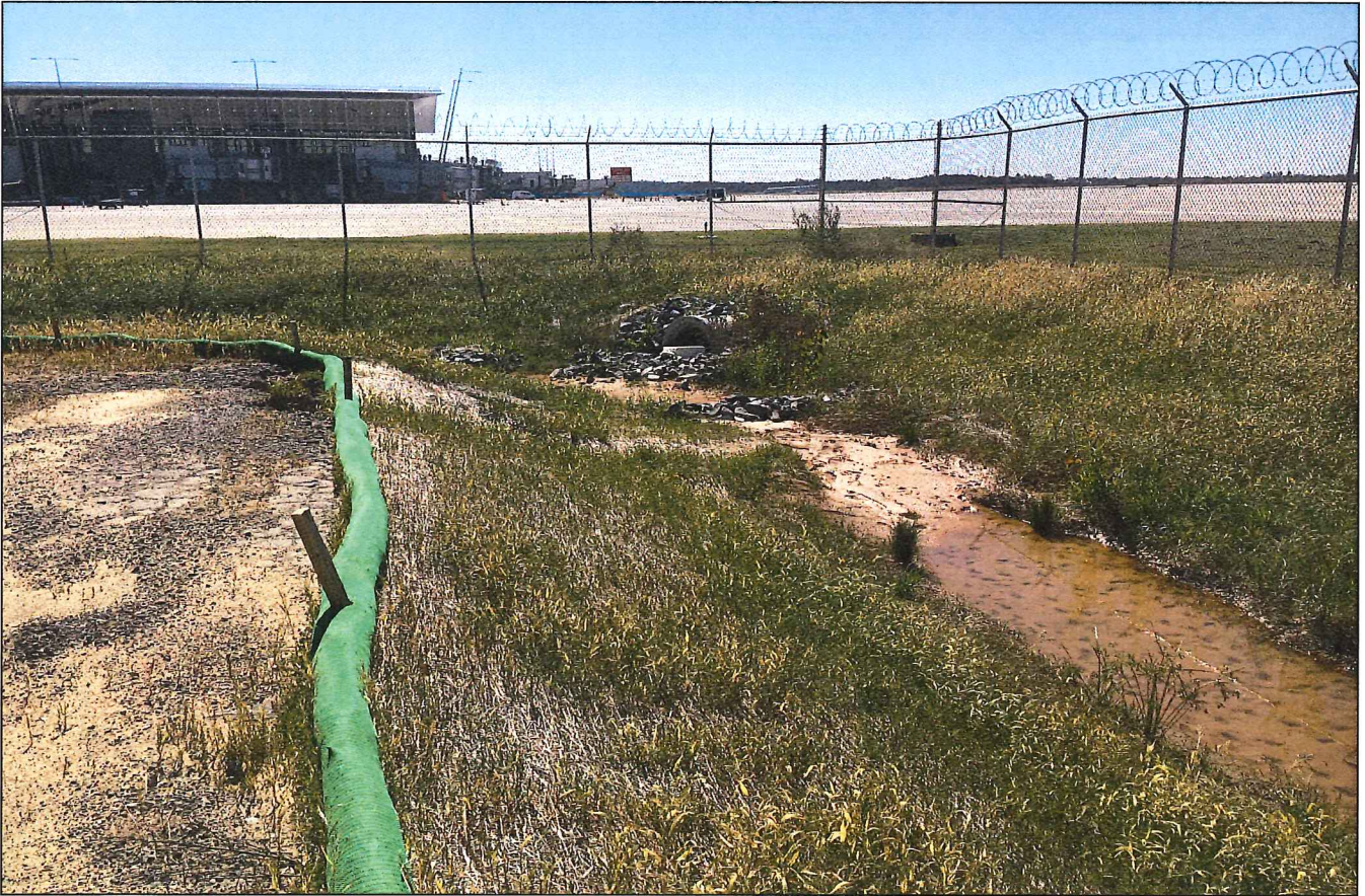
Photograph location E2: Non jurisdictional wet weather conveyance, looking south.
