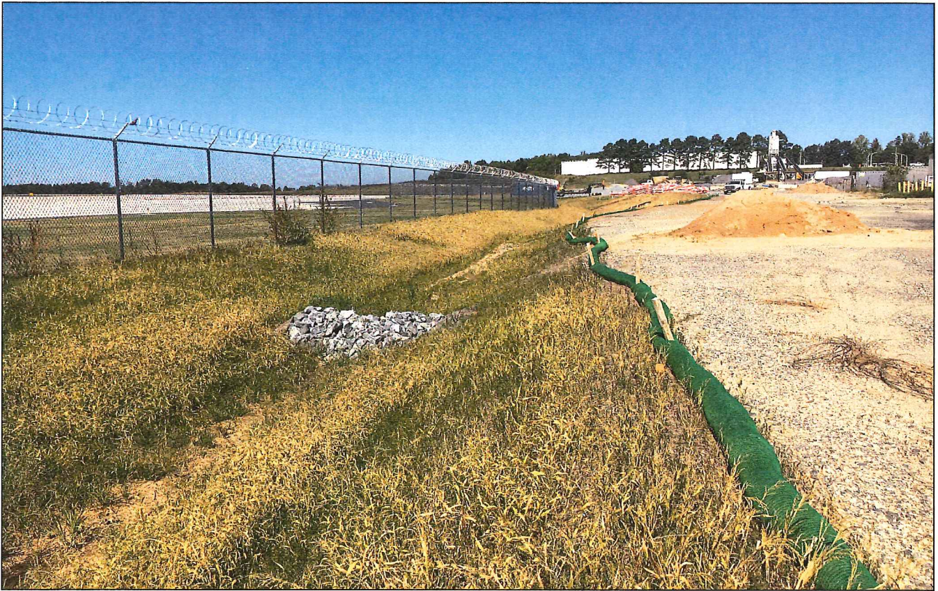
Photograph location E1: Non jurisdictional wet weather conveyance, looking north.
