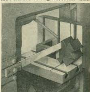
Angle Fixture on Blocking Out Job
