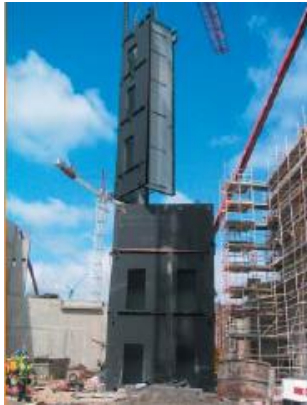
Figure 2-35 Dundrum Cinema Lift Core, Corus (2004)
