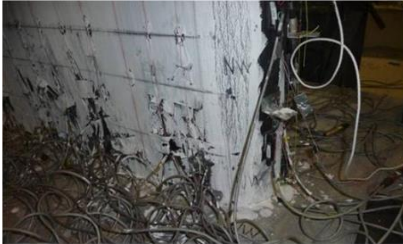
Figure 5-3 North West View for Specimen CFSSP-NB1 at 0.6% Drift
