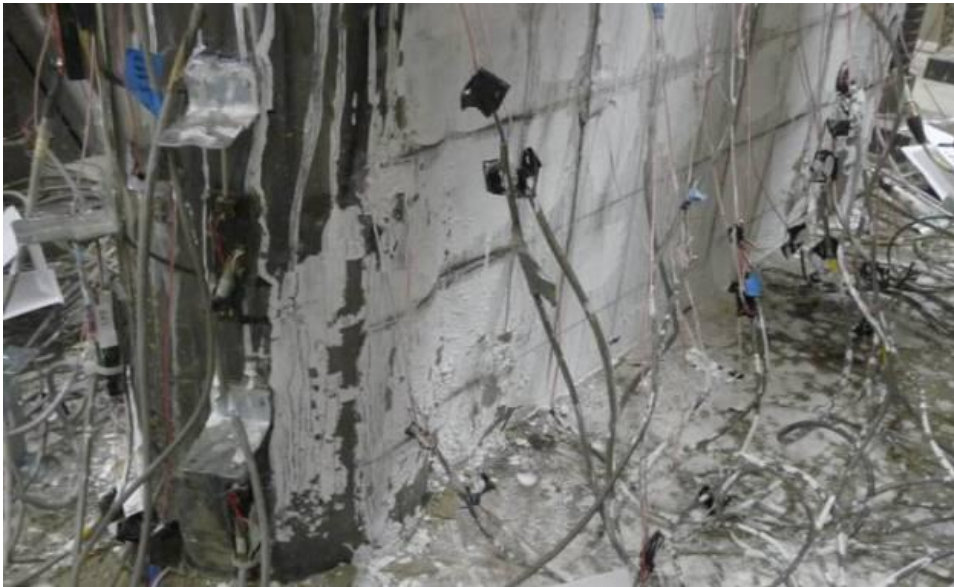
Figure 5-54 Onset of Local Buckling for Specimen CFSSP-B2 at 2% Drift
