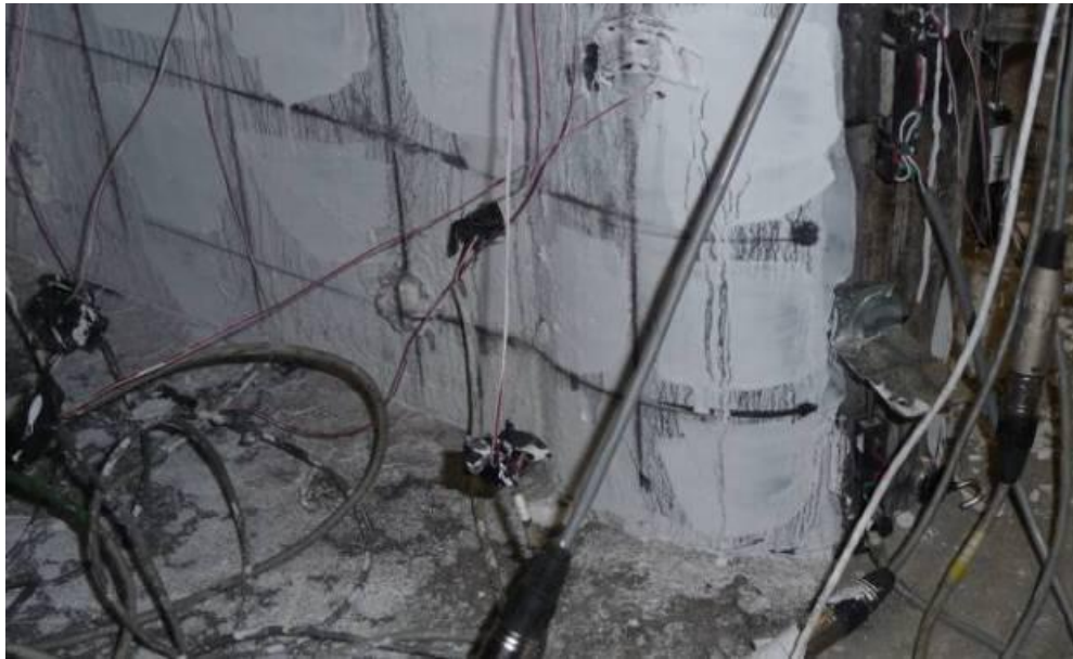
Figure 5-52 South West View Specimen CFSSP-B2 at 1% Drift
