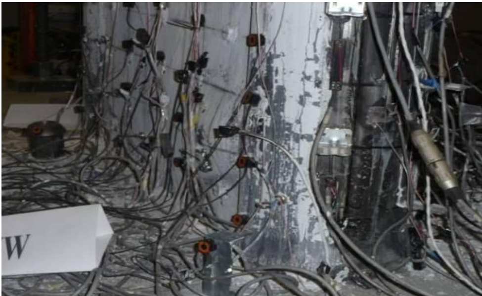
Figure 5-58 South West View Specimen CFSSP-B2 at 3.33% Drift
