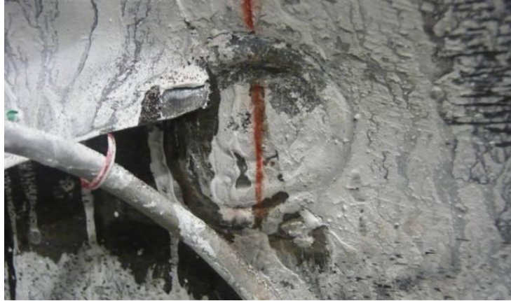
Figure 5-11 Specimen CFSSP-NB1 Tie Bars Plug Welding Cracks Near Mid Cross-section at 2.4% Drift
