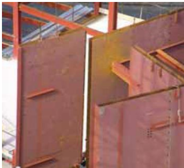
a) The Steel Panel Forming the Bi-Steel Product
