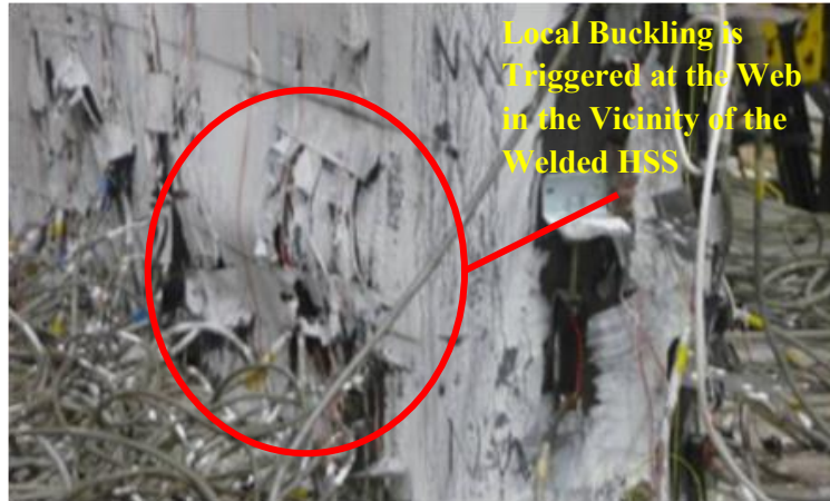
Figure 5-6 North West View for Specimen CFSSP-NB1 at 1.8% Drift
