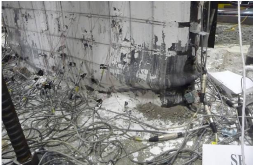
Figure 5-34 Crushed Concrete Debris Spalling from Cracked Skin of CFSSP-NB2 at 3.6% Drift
