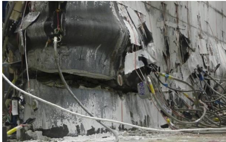
Figure 5-17 Fracture of the CFSSP-NB1 Specimen East Side at 3.6% Drift
