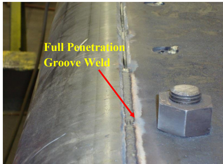
Figure 4-19 Welding between Half HSS and Steel Web Plate
