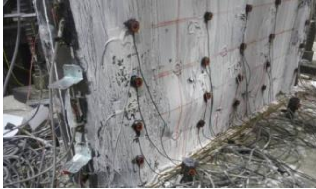
Figure 5-41 Local Buckling of Web Plate for Specimen CFSSP-B1 at 2% Drift
