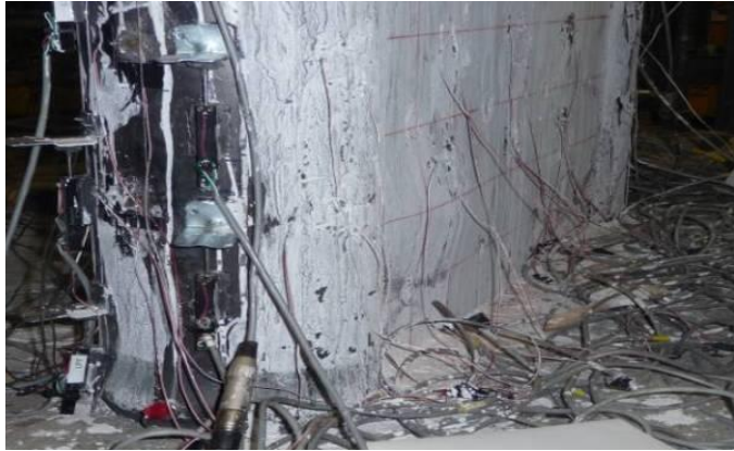
Figure 5-43 Local Buckling of the HSS in Specimen CFSSP-B1 at 2.67% Drift
