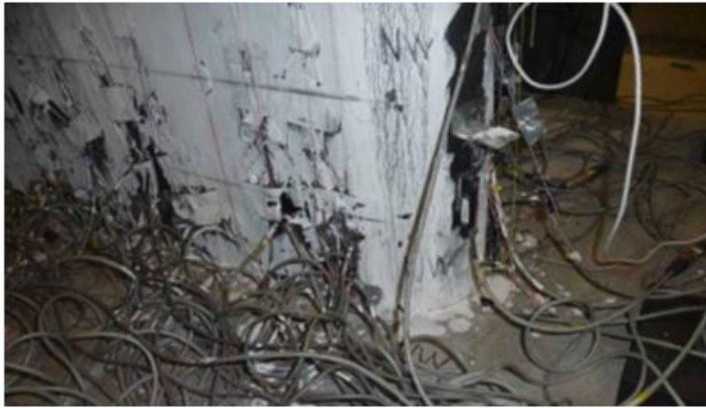
Figure 5-4 North West View for Specimen CFSSP-NB1 at 0.9% Drift
