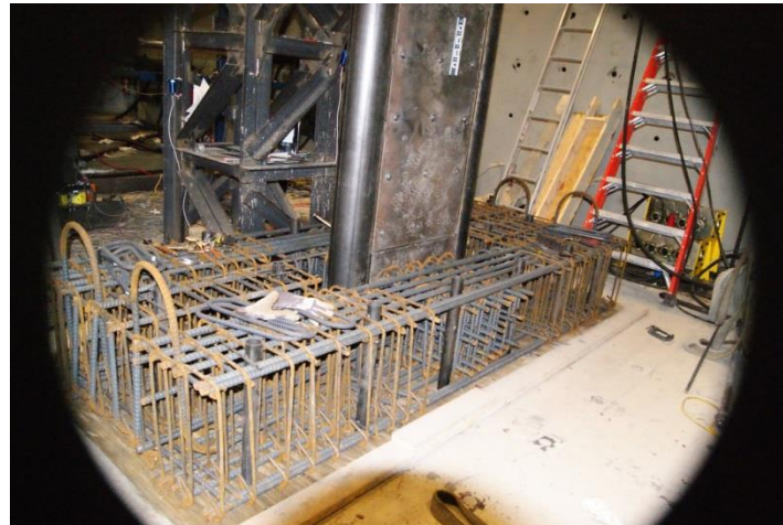
Figure 4-26 Final Assembly for the Foundation Re-bars
