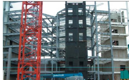
Figure 2-35 Dundrum Cinema Lift Core, Corus (2004)
