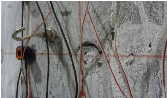
Figure 5-42 Half Diameter Fracture of Tie Bars Plug Welding of CFSSP-B1 at 2% Drift
