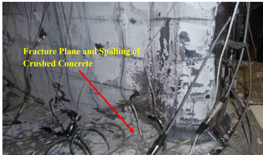
Figure 5-62 Spalling of Crushed Concrete in Specimen CFSSP-B2 at 4% Drift
