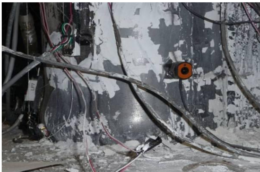
Figure 5-56 HSS Local Buckling in Specimen CFSSP-B2 at 2.67% Drift
