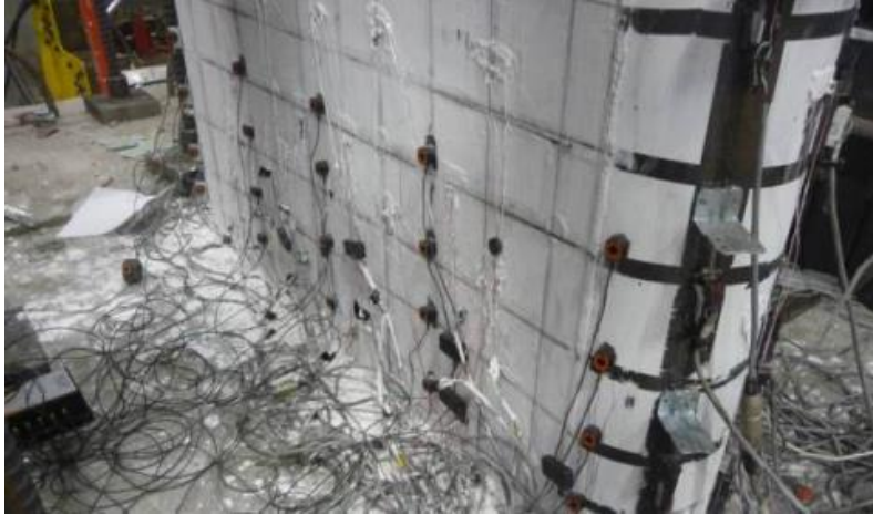
Figure 5-21 North west View for Specimen CFSSP-NB2 at 0.6% Drift
