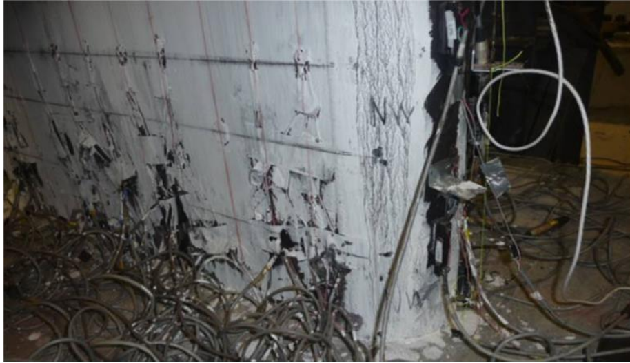
Figure 5-2 North West View for Specimen CFSSP-NB1 at 0.4% Drift
