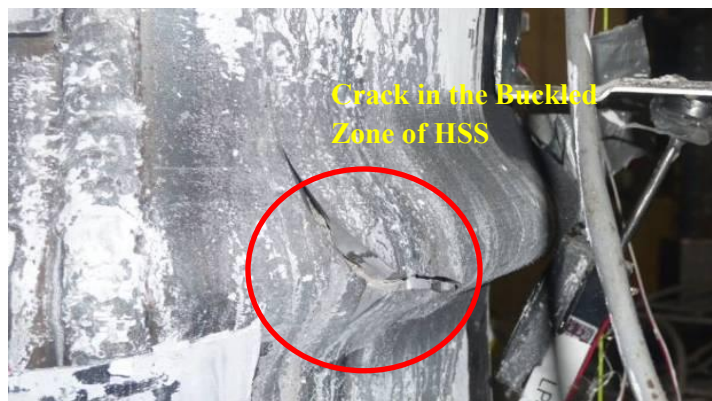
Figure 5-15 First Crack in the HSS Part of the CFSSP-NB1 at West side at 3.6% Drift
