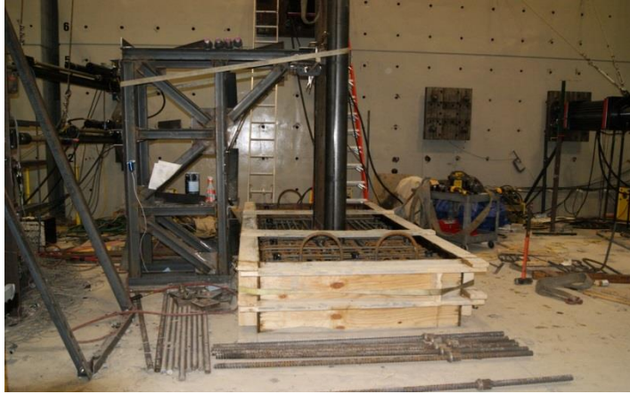
Figure 4-27 Shoring of Specimen Preparing for Concrete Pouring
