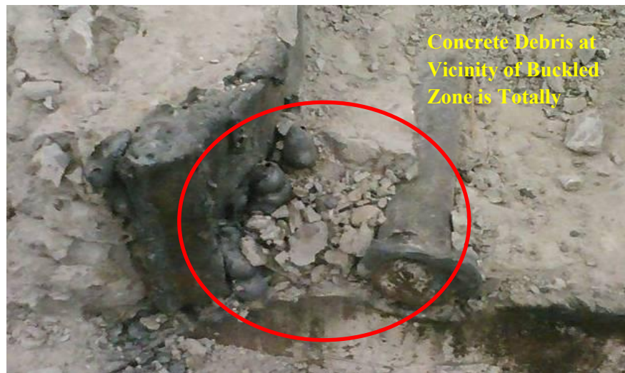
Figure 5-50 Condition of Concrete in the Buckled Zone of Specimen CFSSP-B1
