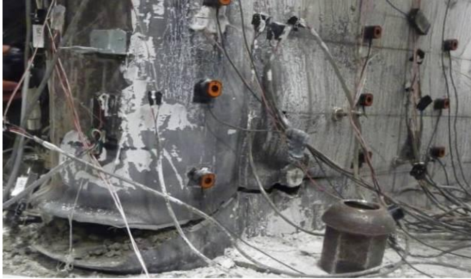
Figure 5-65 Base Fracture of Specimen CFSSP-B2 at 4.67% Drift
