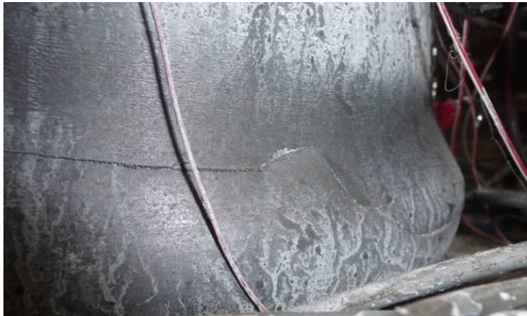
Figure 5-48 Fracture of the HSS Portion of Specimen CFSSP-B1 at 4% Drift
