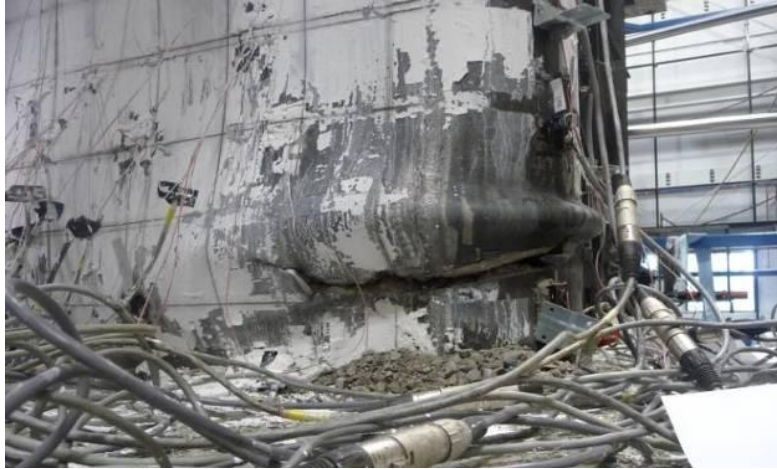
Figure 5-35 Fracture of Specimen CFSSP-NB2 at 4.2% Drift
