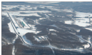
Toyokoro Proving Ground (completed 1992) Location: Toyokoro-cho, Nakagawa-gun, Hokkaido Area: approx. 7,480,000 m 2 Total circumference: 7.9 km; Poor road circumference: 15.8 km
