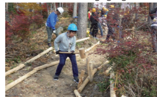
Maintenance of the walking path
