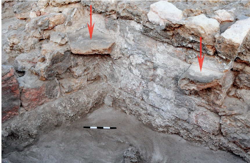
FIG. 19. Two blocks embedded in the southern wall of the pylon of the Ptolemaic gate, above the well located inside the gate chamber, view looking northwest; the blocks probably supported a wooden floor or cover above the well; scale = 50 cm (S. Sidebotham, modified by S. Popławski).
