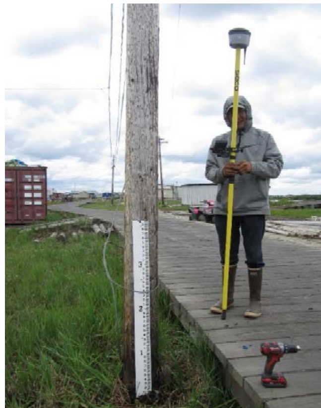
Figure 3: Emmett Matthias installing tide staff (Pollock 2017).
