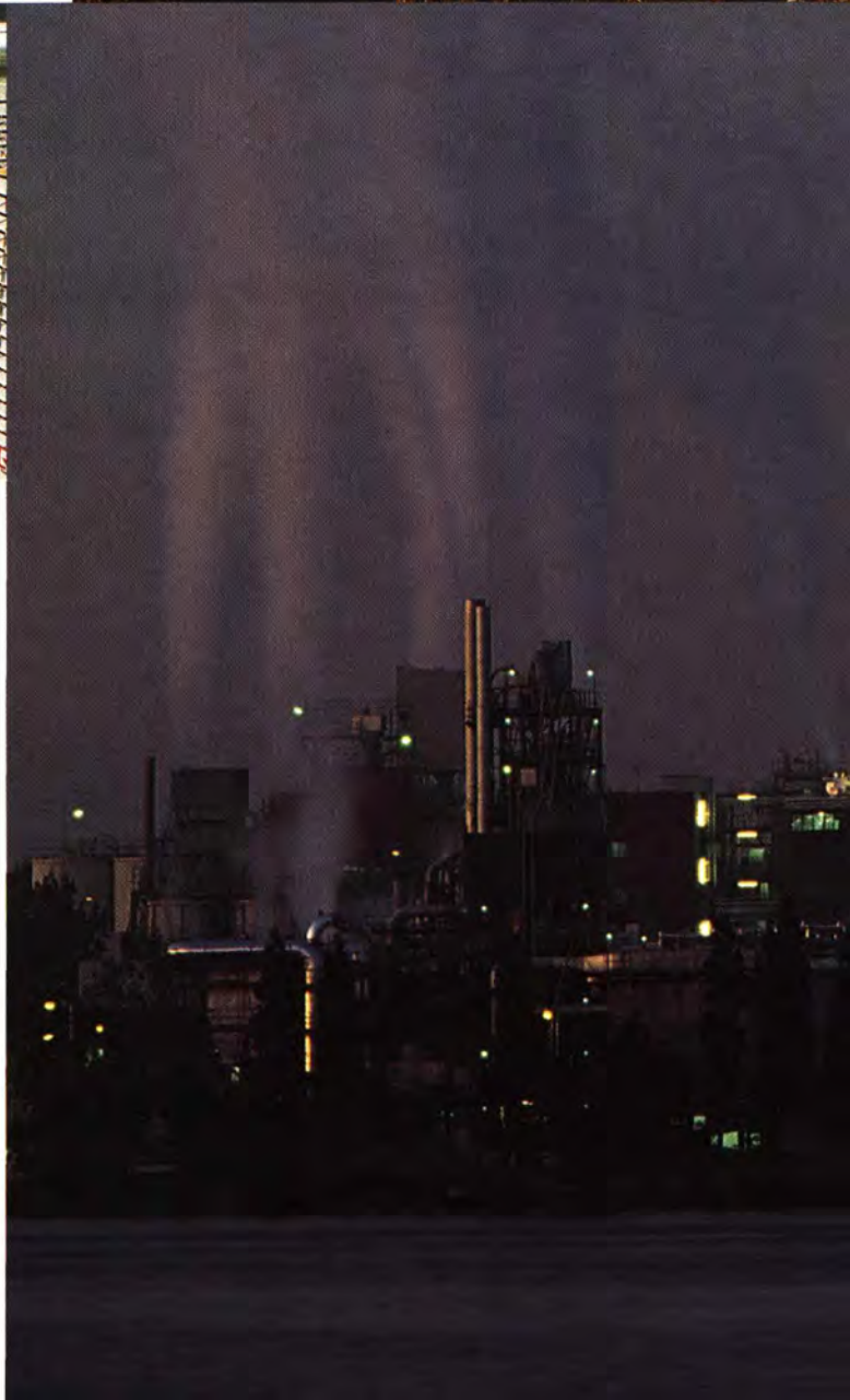
Amsterdam. Production facilities for refinery catalysts and thermoset intermediates.
