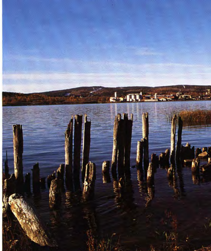
Sundsvall, Sweden. Multipurpose plant for specialty chemicals and industrial products.
