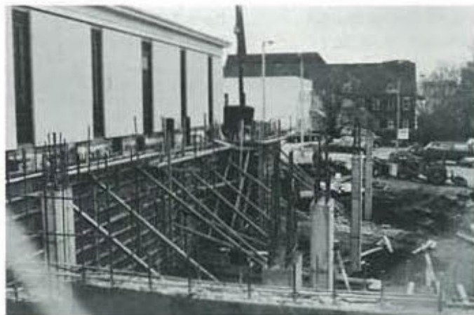
November 1990: The underground parking facility takes shape.
